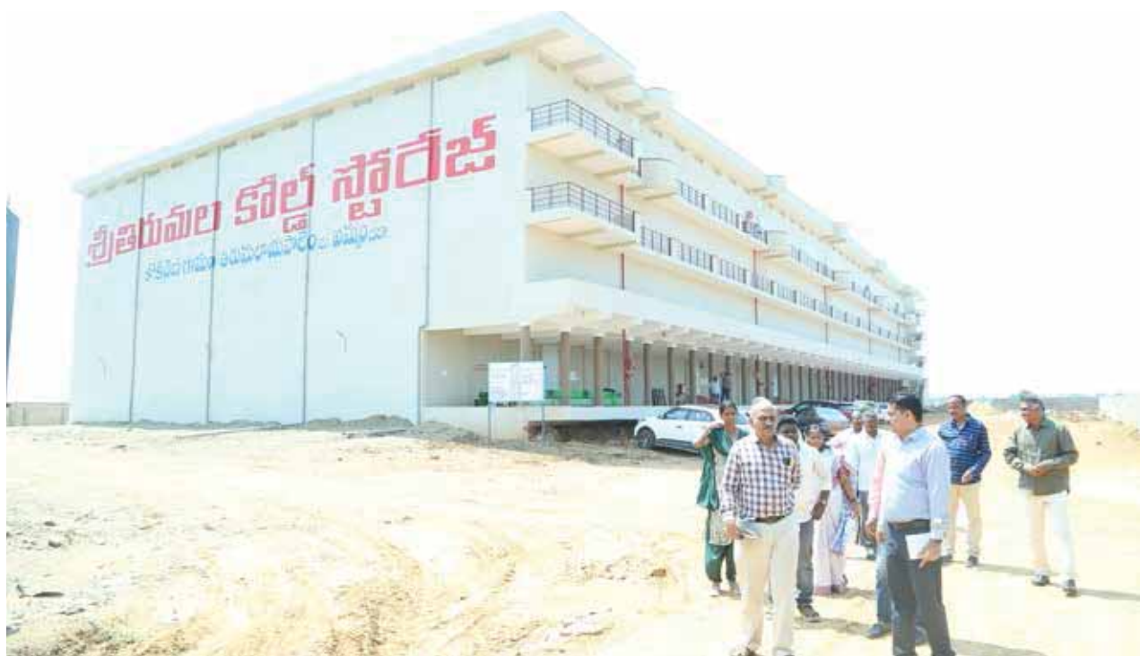
NHB assisted Cold Storage project at Telangana
